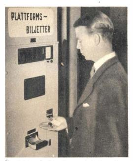
Installed in a Swedish railway terminal, this machine not only issues train tickets and change upon insertion of coins in slots, but also snaps a photo of persons passing slugs.
