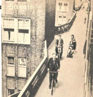
Double-decker streets like this one are being tested in Rotterdam, Holland. Two stories above ground level, the novel streets are supported by attachment to nearby buildings.
