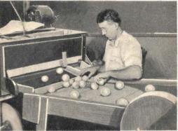
Peaches fed to a conveyor belt of this sorting machine (top) pass through a series of brushes that "shave" the fuzz off, after which peaches are selected for size and grade (bottom).
